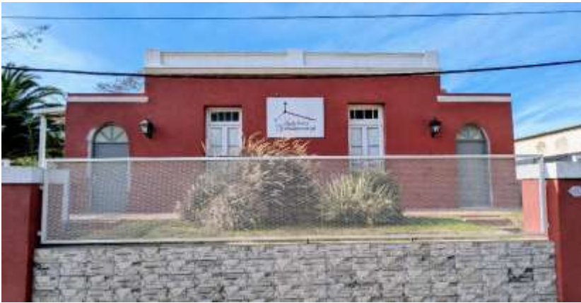
The building is really taking shape, inside and out!
